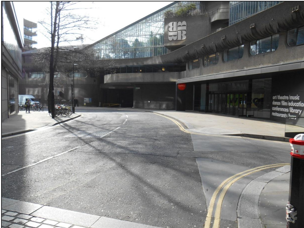
Barbican Centre entrance – before
